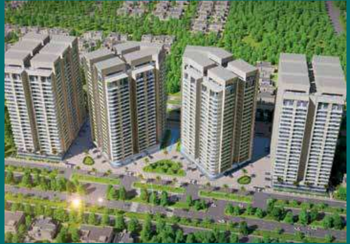
Residential high rise towers in DHA Lahore phase VI featuring world class amenities and comfort
